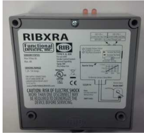
Figure 20: Flow Proving Device
